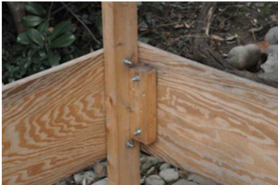
Securing Panels with Machine Bolts
